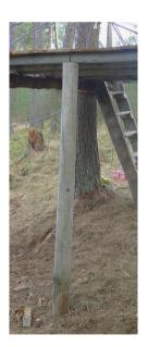
The widest gap between the trees was causing a cross-beam to flex so we added a supporting leg to make it stable.
